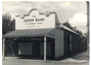
Union Bank 225 Whitehorse Rd Balwyn, nd. Reproduced with permission of Australia and New Zealand Banking Group Limited (UH3-125)
