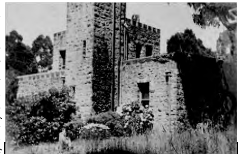
May Reid's retreat Glenleven , Olinda, is known locally as 'The Castle'. A big garden surrounds it. It was designed with a large central music room or hall with bedrooms and other rooms around each side.
