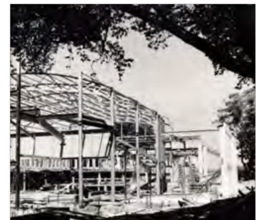
Building the Camberwell Civic Centre CHS 0000-56-6
