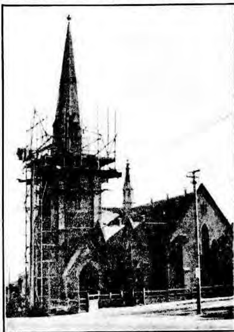
Trinity Presbyterian Church, Riversdale road, Camberwell, now has a new spire, which has been erected in memory of the 30 years of service of the Rev. P. J. Murdoch at Camberwell. A dedicatory service will be held in the church on June 13.
