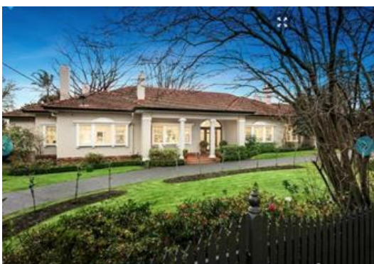
Left: The Victoria Avenue, Canterbury house before demolition in January 2018
